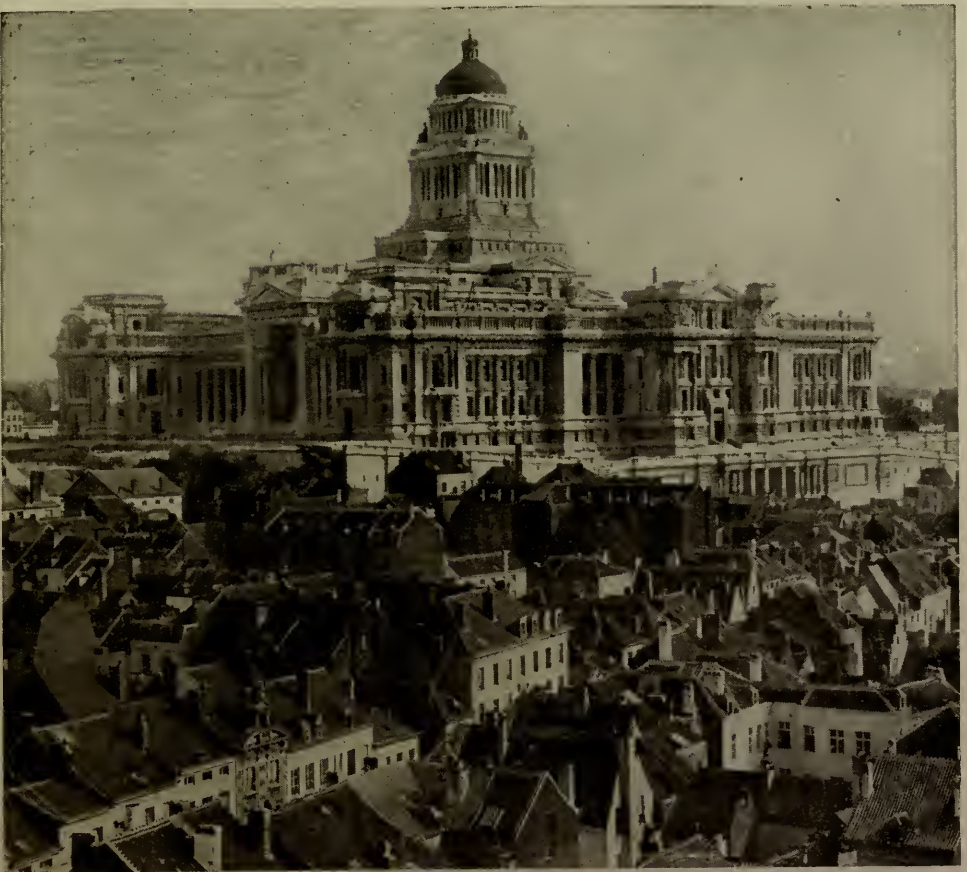
THE BRUSSELS PALAIS DE JUSTICE; ONE OF THE WORLD'S LARGEST BUILDINGS
