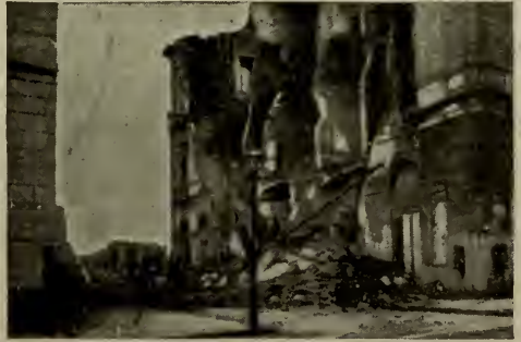
THE DAMAGED POST-OFFICE
