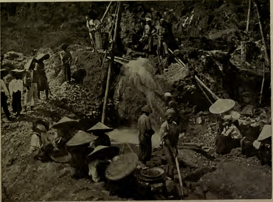
CRUDE NATIVE METHOD OF WASHING THE RUBY-LADEN GRAVEL
