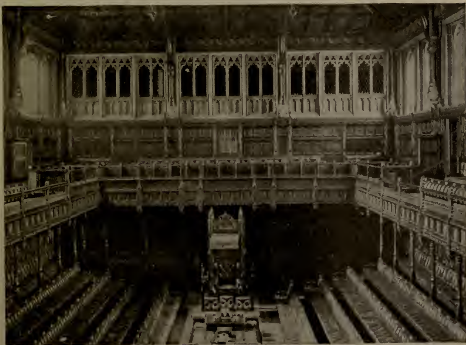
INTERIOR OF THE HOUSE, LOOKING TOWARDS THE SPEAKER'S CHAIR
