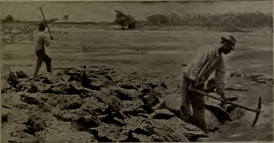
NATIVES DIGGING THE PITCH
