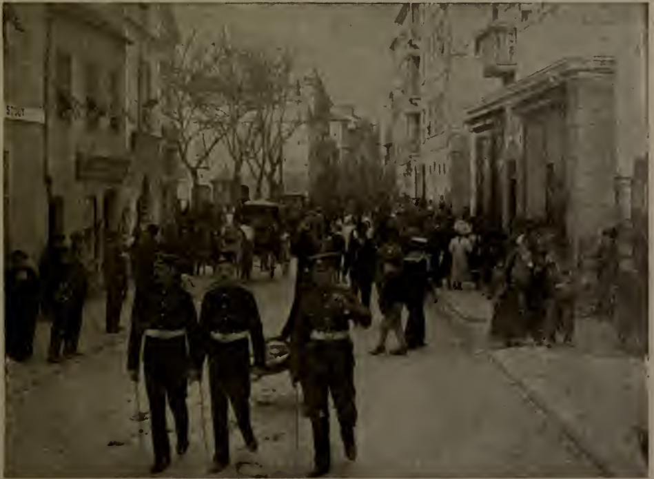
WATERPORT STREET, THE PRINCIPAL BUSINESS THOROUGHFARE
